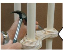
Drive in the nails and countersink with a nail punch. Fill the holes with a dab of wood filler. (fig. 4s)
