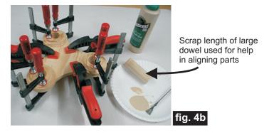
Glue together the feet parts and the three 0.25" dia. x 2" wood dowels. Use the scrap length of the large diameter dowel to help align the parts. Clamp until
