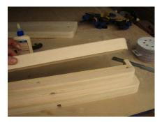
Start gluing the shelf together piece by piece. The three back pieces should all be flush on the top side.
