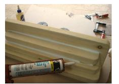
For this example the edges of the boards were routed with a 1/2" roundover. So a caulk line is being installed in the inside corners to be smoothed round to match the routed edge.
