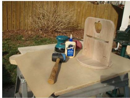
Glue the base to the center piece. A rubber mallet might be needed to push the center piece into the base piece.
