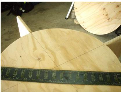
Using a straightedge draw lines from the center of one leg to the center of the next. You are creating a layout line to run screws in, it can just be eyeballed.
