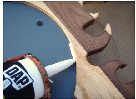
Drop the mirror into place once the polyurethane has had time to dry. Run a small bead of silicone or caulk around the perimeter of the mirror.
