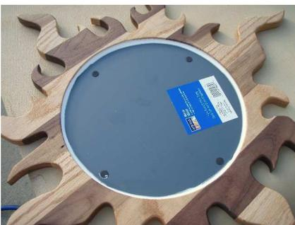
Smooth the caulk into place and allow the caulk to dry with the mirror facing down until it has setup. Depending on the wall surface, select the proper mounting hardware from your local hardware store.
