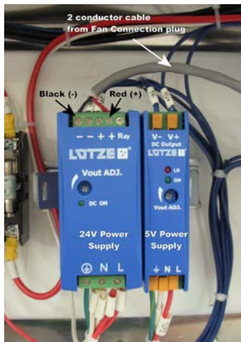
24V power supply for PRS Alpha
